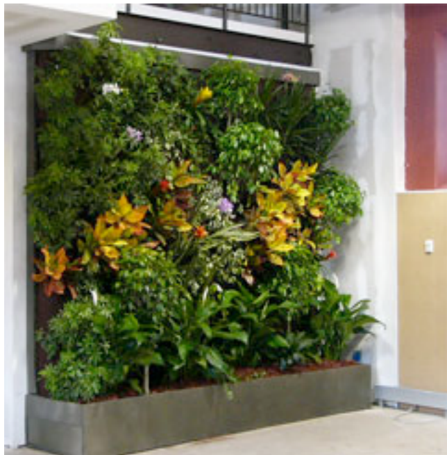
Living Wall installation, Baltimore, MD. This 110 sq ft (10 sq m) wall filters all the air for its 7,500 sf office building.
